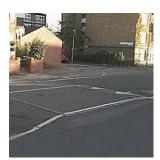
Similar to road humps but longer and with a flattened top, sometimes used to give pedestrians a level crossing between footways. They are especially useful where there are a lot of pedestrians.
