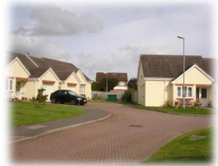
The walls are painted render with a traditional dual pitched roof and concrete tiles. Some of the properties have chimneys and dormer windows. The doors and windows are white uPVC with bricks above.
