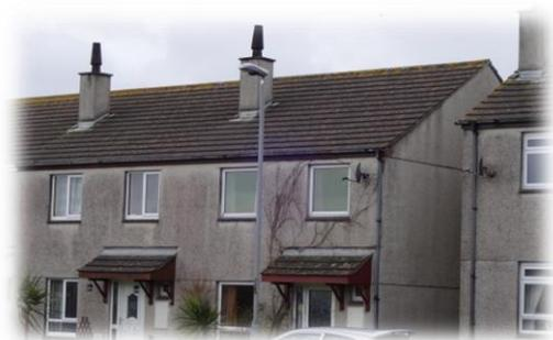
The roofs are dual pitched with concrete tiles and chimneys. The walls are pebble dashed grey and the windows and doors are white uPVC. The porches have canopies and some with a built in porch.
