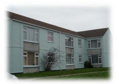
Some of the properties have conservatories to the rear. The roofs are dual pitched with concrete tiles and chimneys and one property has solar panels. The walls are painted render with uPVC or aluminium windows and uPVC doors. The front gardens are mainly open plan with soft landscaping, and a couple have been fenced or have hedging. The rear gardens are enclosed and some properties have conservatories.
